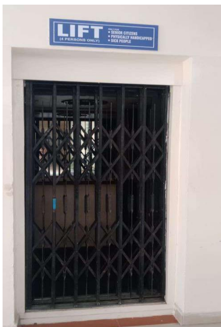
Block-AB Lift for G+ 3Floors
