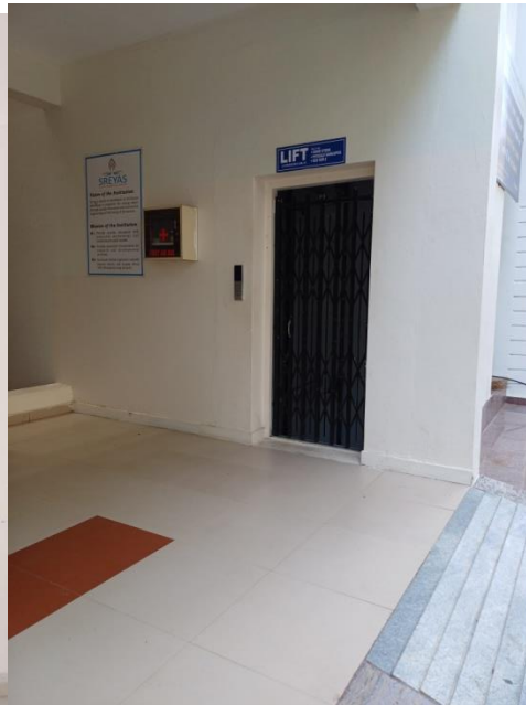
Block-C Lift for G+ 3Floors
