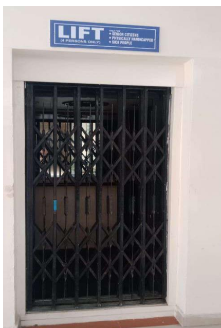
Block-AB Lift for G+ 3Floors
